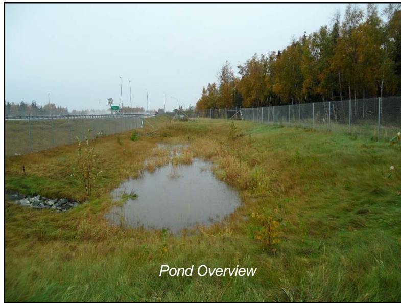
Figure 7: NSH Infiltration Basin September 22, 2016
