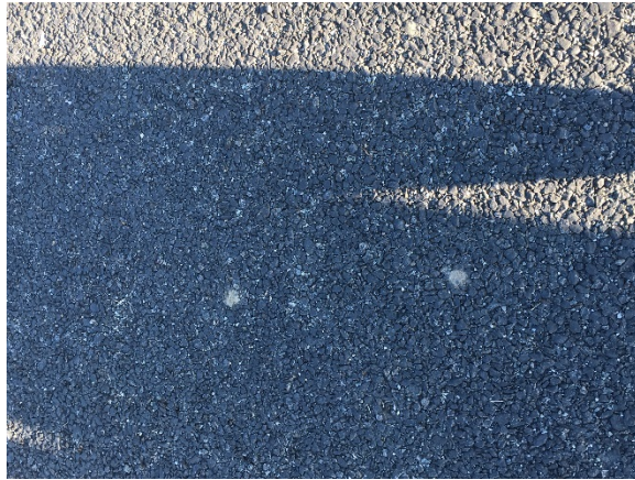
Sand in the Porous Asphalt Pores
