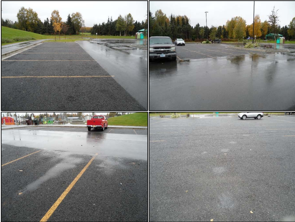
Figure 5: RJSP Parking Lot September 22, 2016
